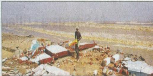
A man looks at his damaged house in Podampeta village
